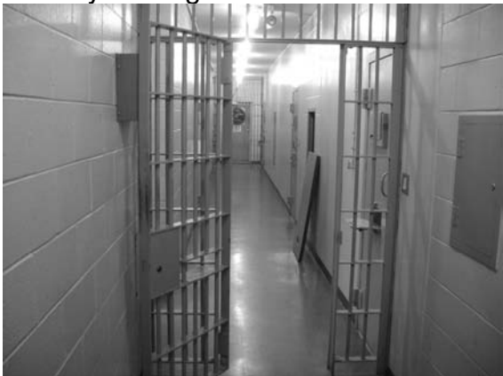
Main jail corridor, cell entrances on left and right.
